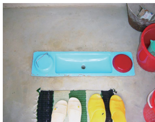
Figure 4. Inner view of toilet. (Taken by the author)
