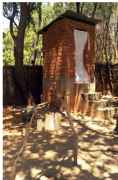
Figure 6. Ecosan toilet constructed by the NICCO Malawi Ecosan project. (Taken by the author)
