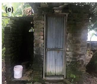
(e) An improved toilet and a hand washing station (bucket) at a village in Tanzania.
