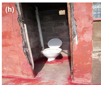
(h) A common improved pour flush toilet at a peri-urban area in Zambia.
