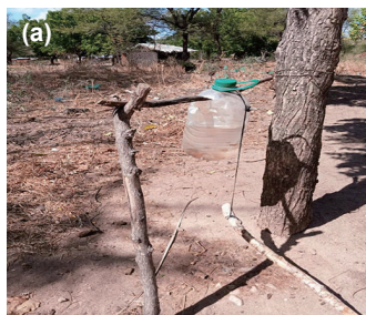
(a) A basic latrine at a village in Malawi with a hand washing station (bottle) installed a few metres from the toilet.
